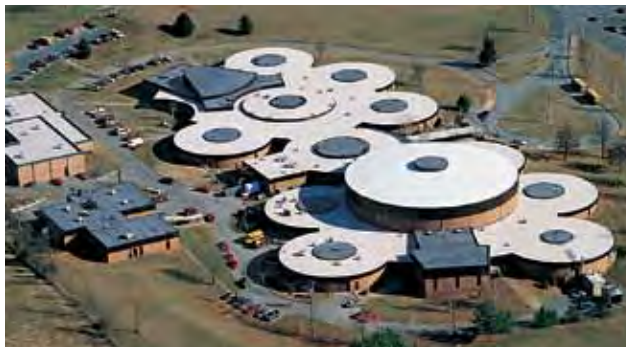
The development of complementary technologies has allowed EPDM to be beneficial in a wide number of applications, including plaza decks and larger projects using white EPDM membrane. Pictured (above) is a plaza deck paver system installed over a 145-mil EPDM system and (below) a white EPDM roof system.
