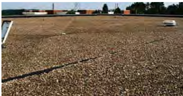
The 29-year-old EPDM roof protecting the Jamerich Building at Northern Michigan University in Marquette, Mich., is still performing well.
